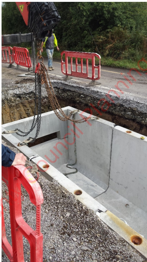
Plate 3-1: Typical Installation and Temporary Reinstatement of Joint Bay
