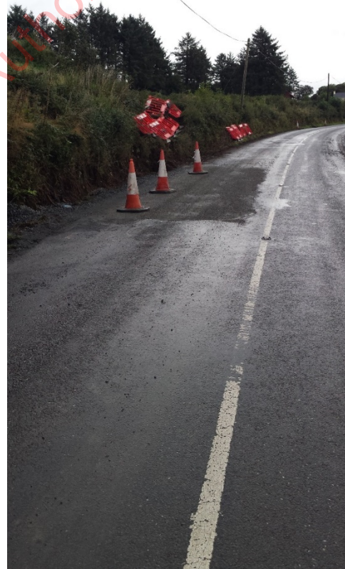
Plate 3-1: Typical Installation and Temporary Reinstatement of Joint Bay
