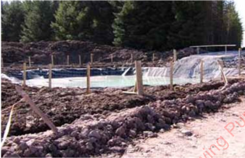
Figure 4-8: Typical Lined Settlement Lagoon for Concrete Washout Facility
