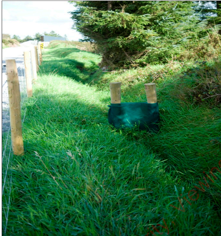
Figure 4-4: Typical Silt Trap across Grassed Swale
