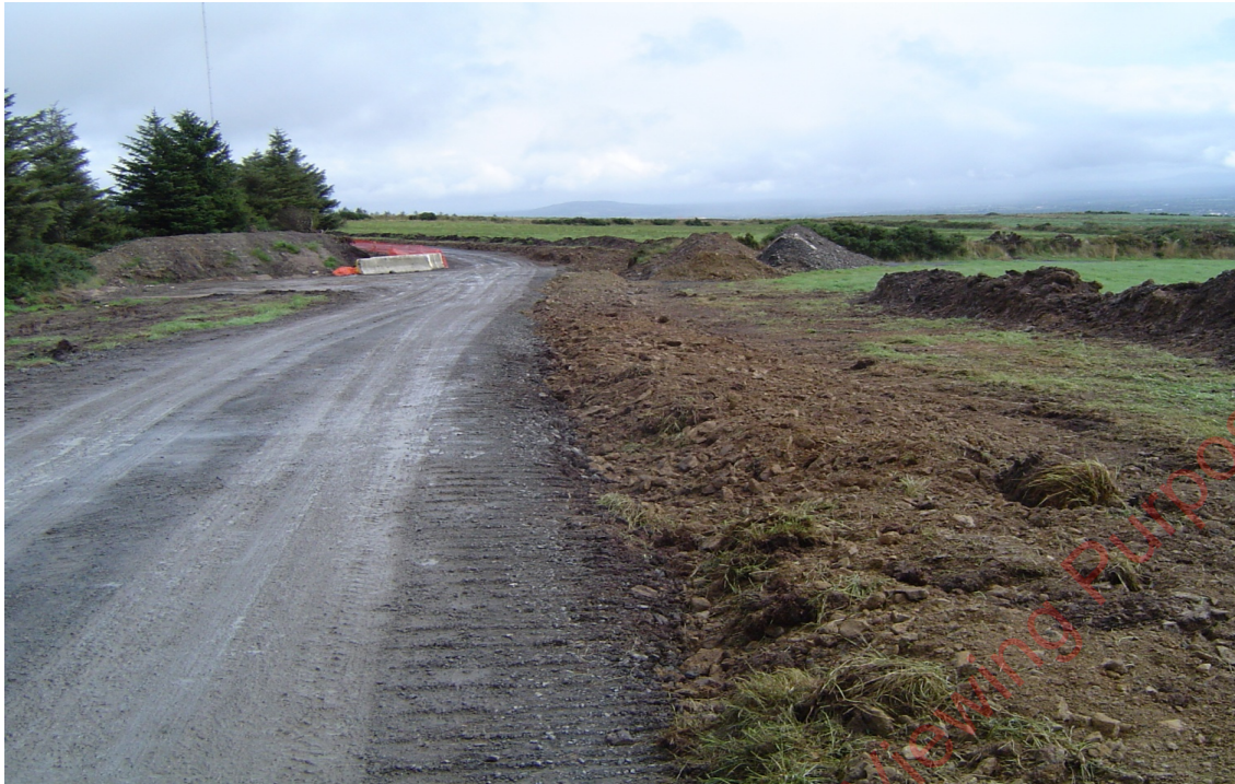
Figure 4-7: Typical Backfill over Cable Trench
