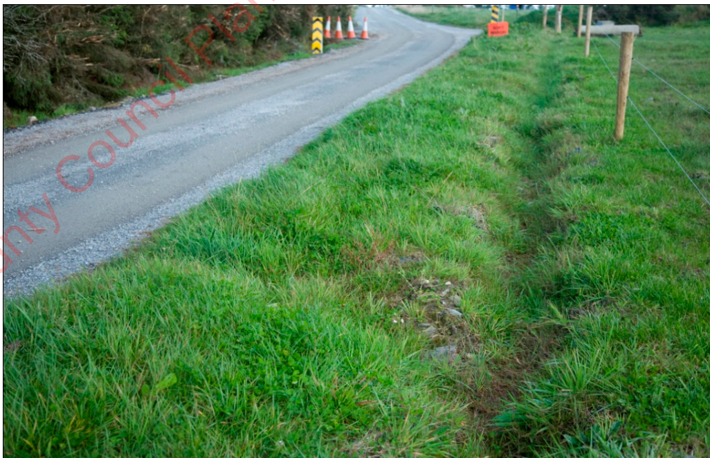
Figure 4-1: Typical Grassed Swale along access track
