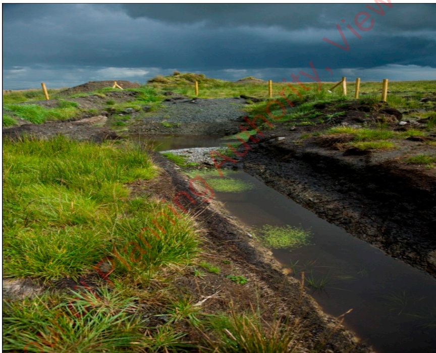
Figure 4-2: Typical Swale draining to Stilling pond
